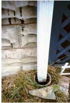
Figure 4-3: Downspout Inflow
