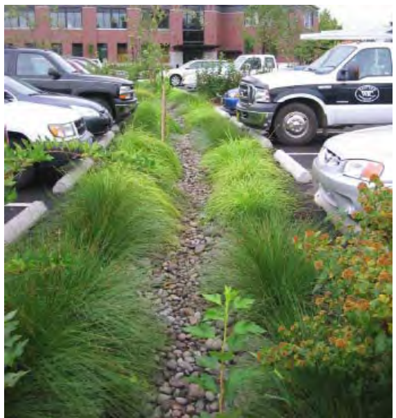
Figure 4-8: Parking Lot Bioretention Islands
