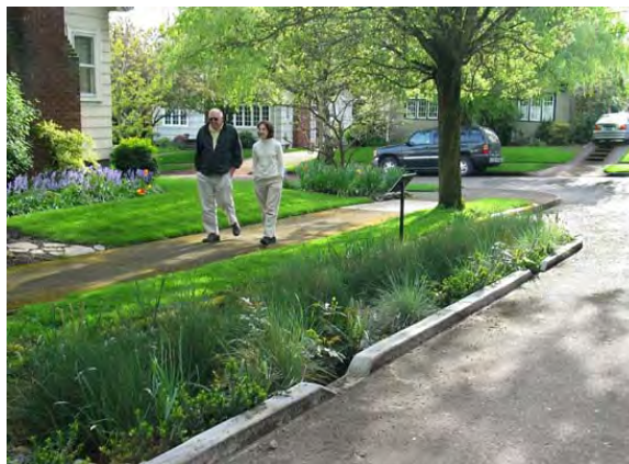
Figure 4-7: Residential Street Bioretention/Green Street
