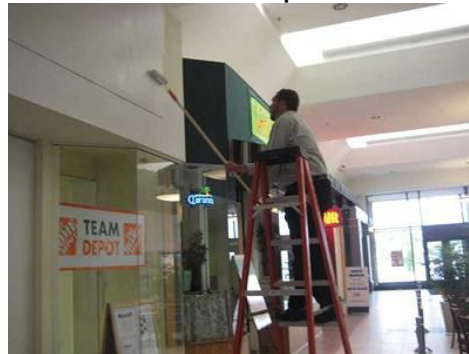
The expansion of the Niles Teen Center was mostly completed June 11 after several days of work from more than a dozen volunteers from Home Depot.
