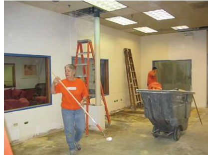
The expansion of the Niles Teen Center was mostly completed June 11 after several days of work from more than a dozen volunteers from Home Depot.
